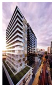
Project: Claremont Manor
